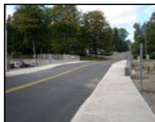
AI provided design and construction inspection services for this Rose Hill Avenue Bridge in Danbury, CT
